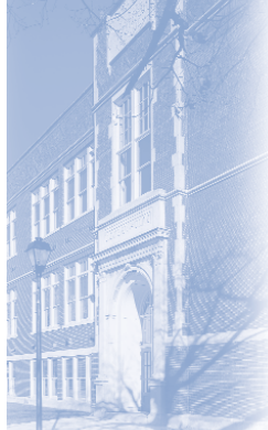
IMG World Headquarters Indianapolis, Indiana
